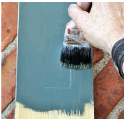
Spread the paint out well in several directions. Finish off following the grain of the wood.
