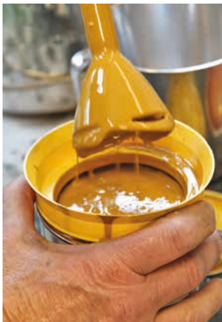
Mix up paint carefully with a hand blender.
