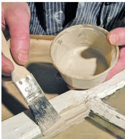
Thinned putty, a simple "delay aging" method.
