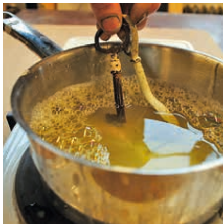
Clean hardware from paint and rust in boiling soap and water.
