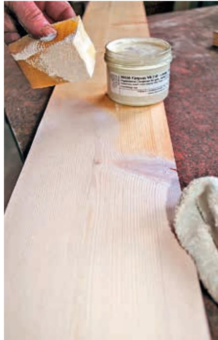
White Linseed Oil Wax on a wooden floor.
