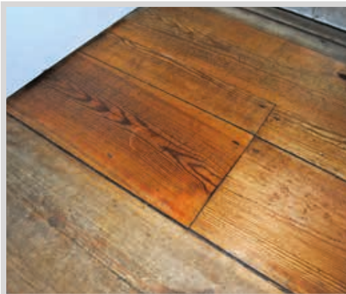
Linseed oil wax before and after.
