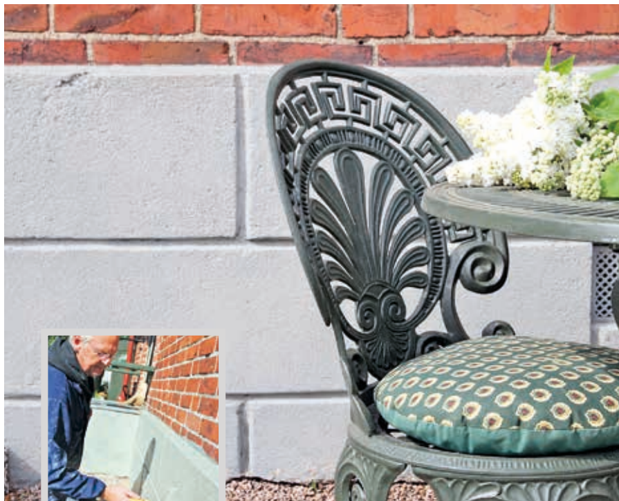
Rendered plinth 20 years after painting. Metal chair painted with Linseed Oil Paint.
